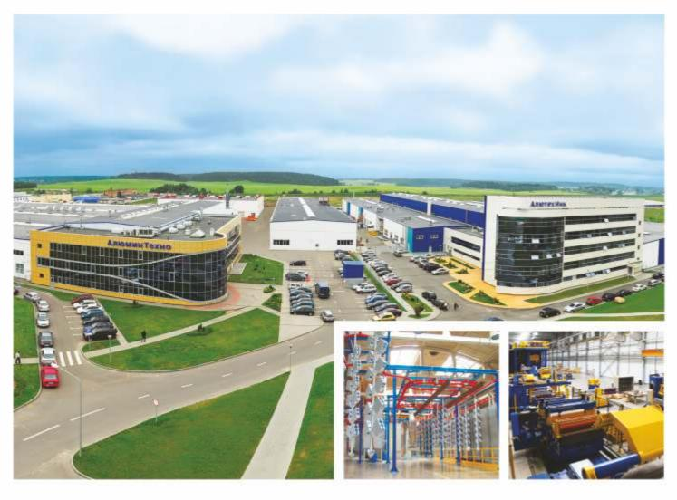
AluminTechno is one of the largest factories in Eastern Europe producing extruded aluminium profiles and performing powder coating and anodic treatment. Factory implements a complete manufacturing cycle, which begins with melting of primary aluminum and ends up with extruded profiles production, their coating and treatment. The plant is fitted with equipment from world's leading manufacturers from the USA, Germany, Italy, Great Britain, Canada and some other countries.
